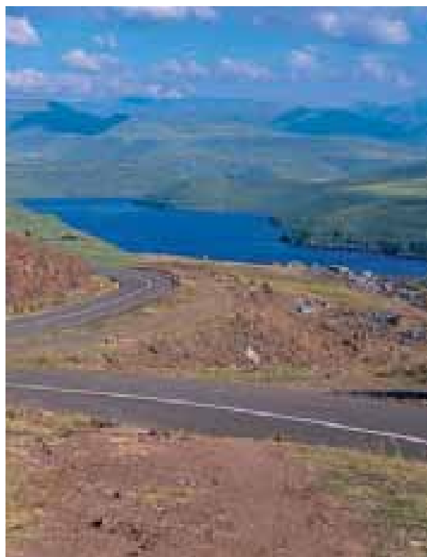
Feeder roads at the Lesotho Highlands water project
